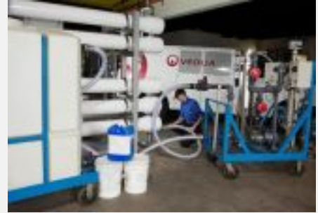
Veolia Team Service performing a Membrane Cleaning on an RO
