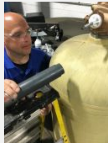
Veolia Team Service performing a Membrane Cleaning on an RO
